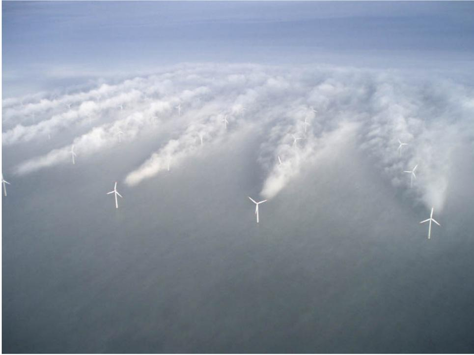
Figure 1: Turbulence patterns revealed by the condensation wake of the Horns Rev 1 offshore windfarm. Photographer Christian Steiness, (Credit: Vattenfall) . <http://ict-aeolus.eu/about.html>
